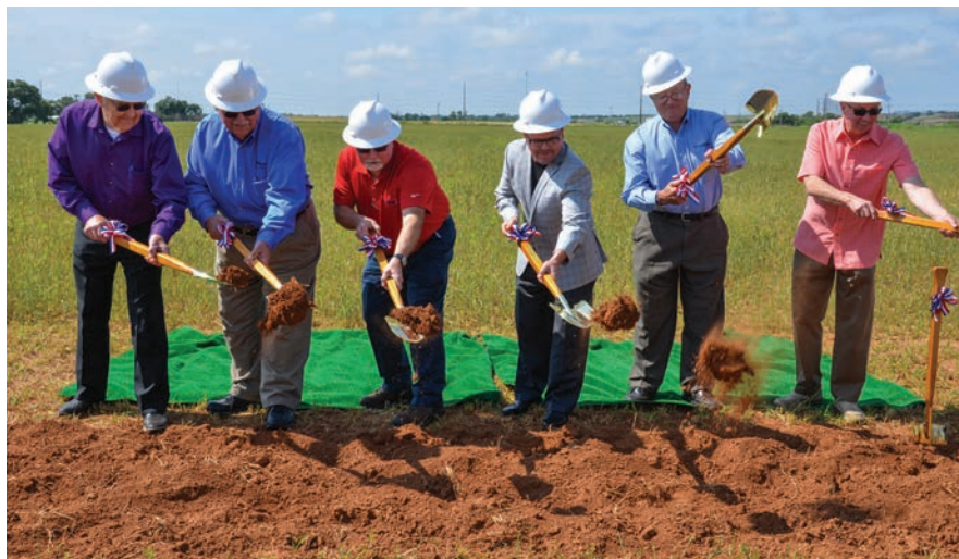
Randy Magnison (red shirt) breaks ground for the new Southern Pioneer Electric Medicine Lodge office in 2015. Southern Pioneer is a not-for-profit wholly-owned subsidiary of Pioneer Electric formed in 2005.
