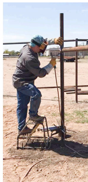
Top: Poles have been set for timed event cattle return pens at the new Ulysses Stampede grounds. Bottom Left: Board Member, Michael Tarbet cuts a saddle into a pipe in preparation to weld it to the post. Bottom Right: Vice President, Wacey Munsell welds the top rail of the new timed event return pens to a post.
