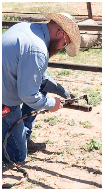
Top: Poles have been set for timed event cattle return pens at the new Ulysses Stampede grounds. Bottom Left: Board Member, Michael Tarbet cuts a saddle into a pipe in preparation to weld it to the post. Bottom Right: Vice President, Wacey Munsell welds the top rail of the new timed event return pens to a post.
