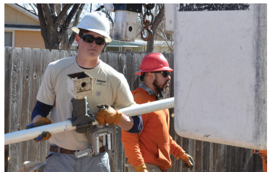
Top: Eric Archuleta makes repairs on section of line in Ulysses. Bottom: Jacob Ogelvie (left) and Abel Diaz (right) start preparing on a job site for a project.
