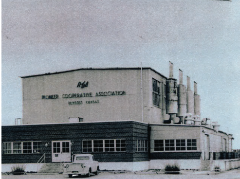
Pioneer Electric's power plant in 1954.
